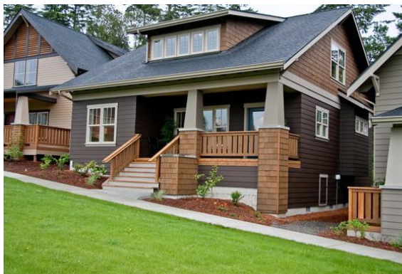
Dormer with a shed roof.
