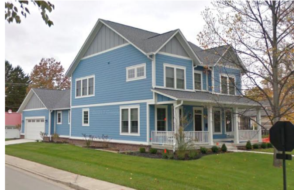
Corner side façade has gable accent and larger, trimmed windows.
