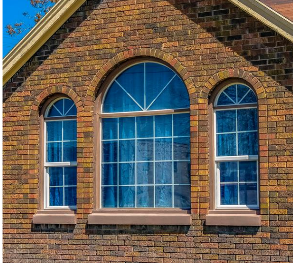
Example of masonry window arch
