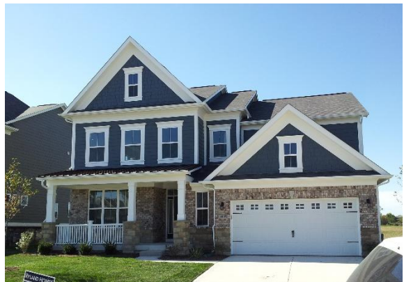
Roof design shows changes in roofline, gables, and a shed roof on the porch.
